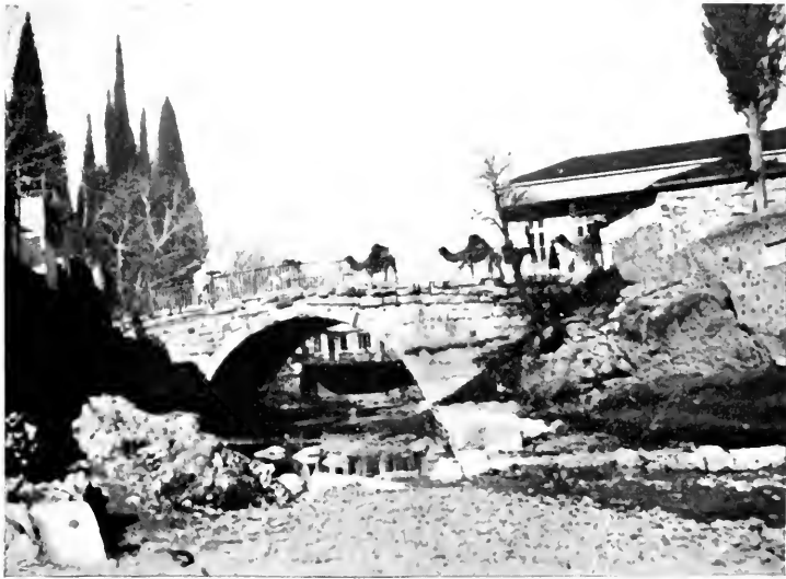
SMYRNA.—The Trade Route entering the City by Caravan Bridge.
